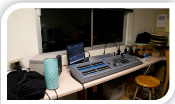
Sound and lighting board
